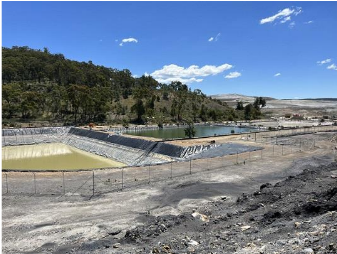
Plate 2 Lined LN Pond 3, 2, 1 (left to right) (Photo taken February 2022)
