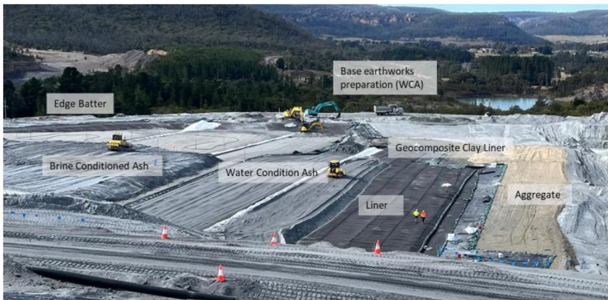
Plate 1 Construction of the Leachate Barrier
