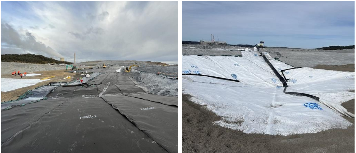
Plate 2 and 3 Leachate Barrier installation and interconnecting drainage pipe work
