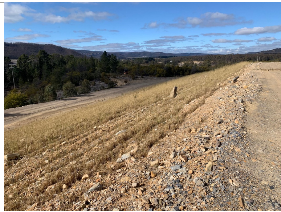
Figure 2 – Revegetation works along north east batter
