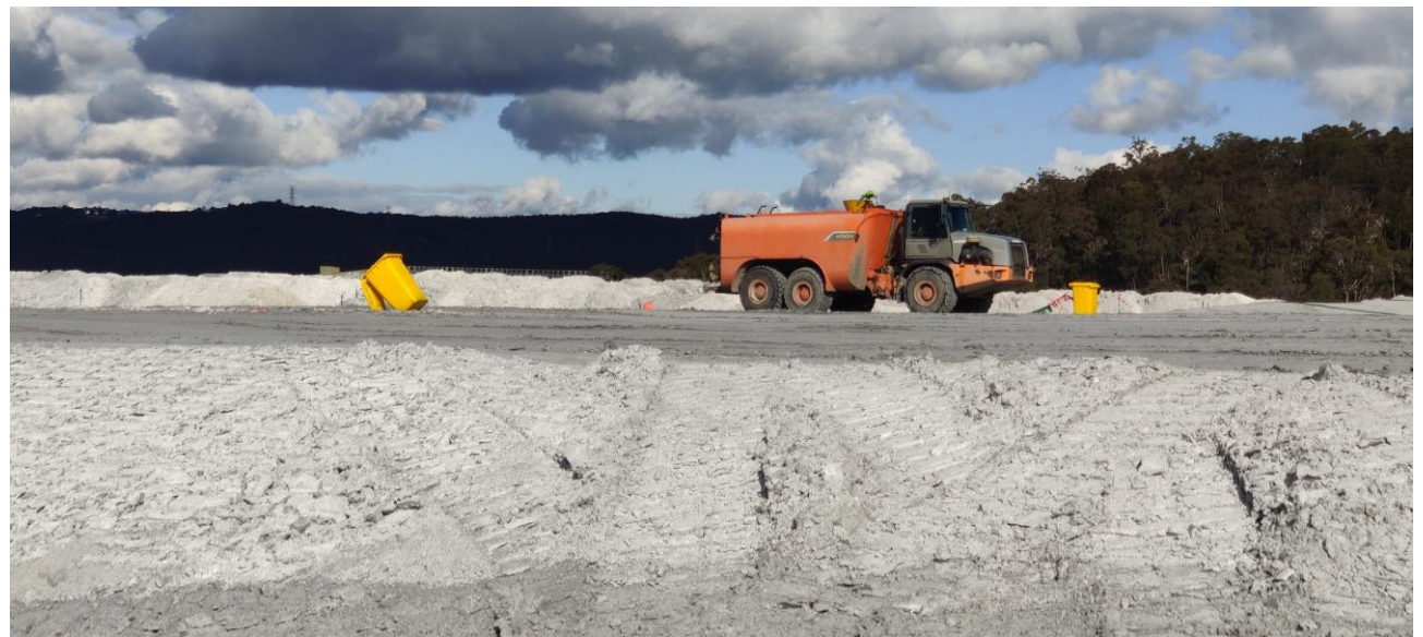
Figure 4b | Photograph of Machinery Operating in Area 1 and Ash Sediment Basin
