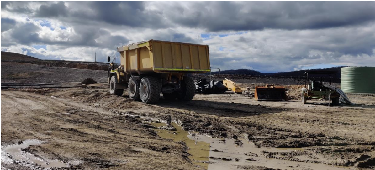
Figure 4a | Photograph of Machinery Operating in Area 1 and Ash Sediment Basin
