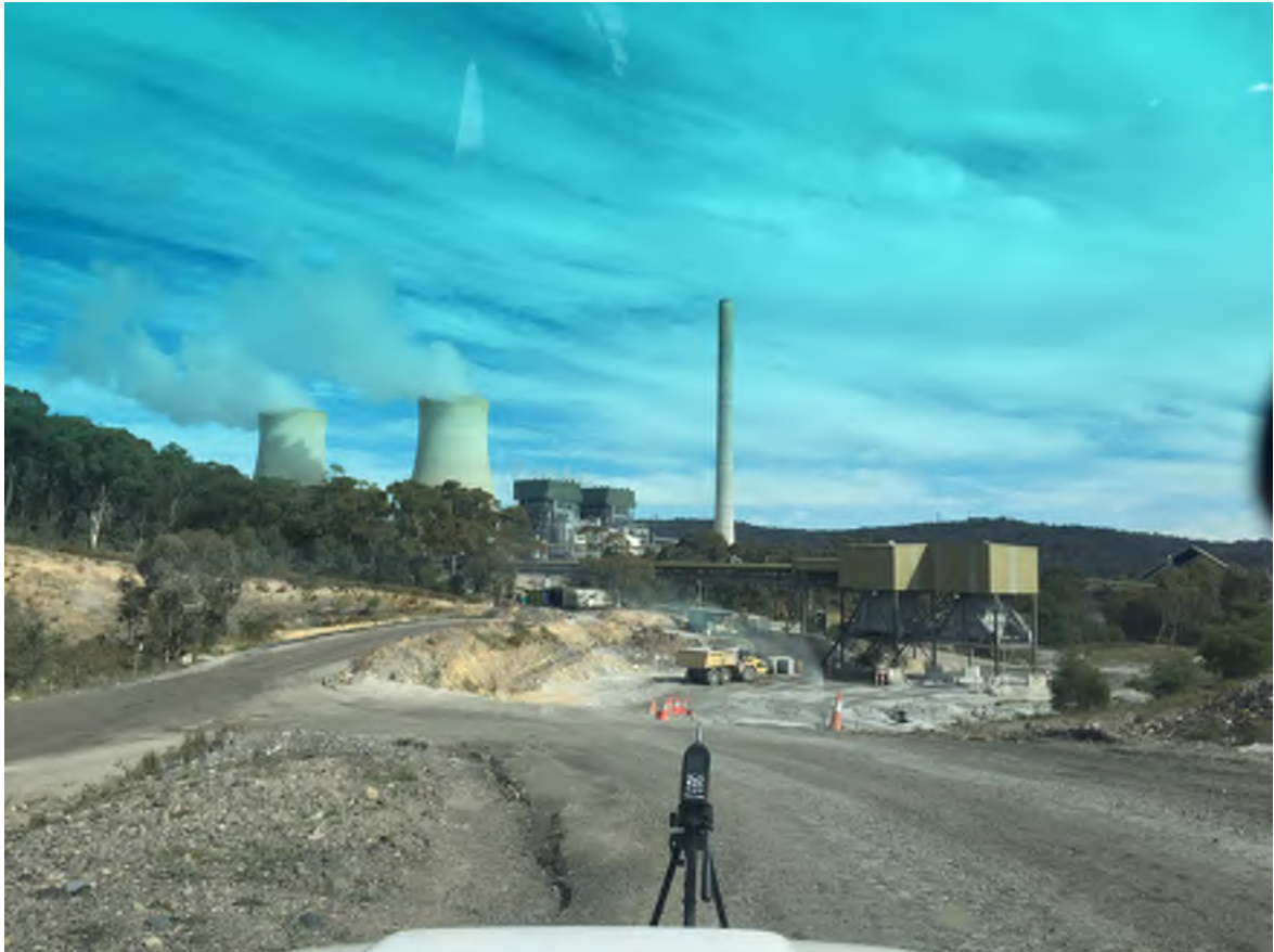
Figure 4 | Photograph of Lamberts North South eastern boundary
