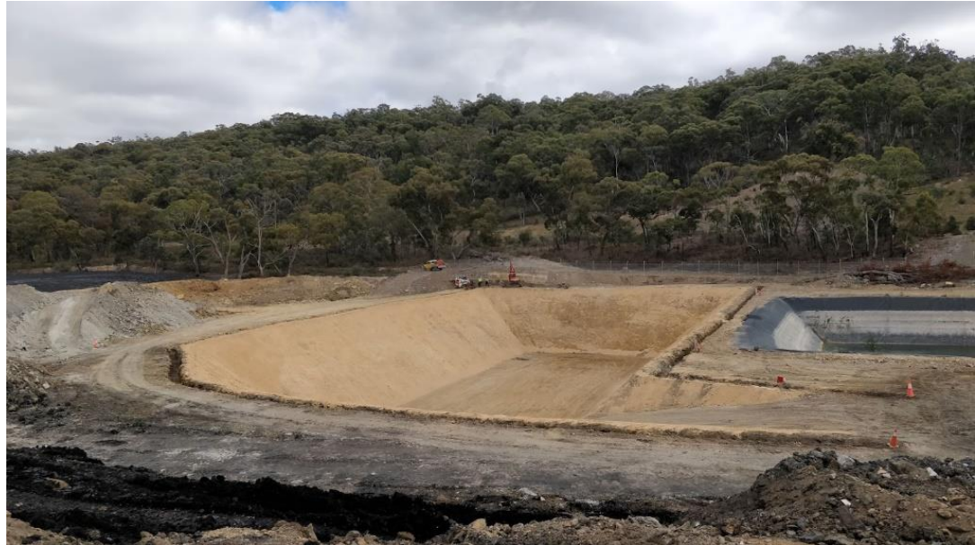
Typical ash placement facility under construction – preparation before laying lining material
