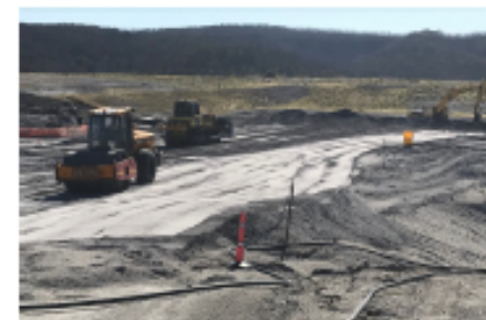
Above: Compaction of ash mixed with water at LNAR
