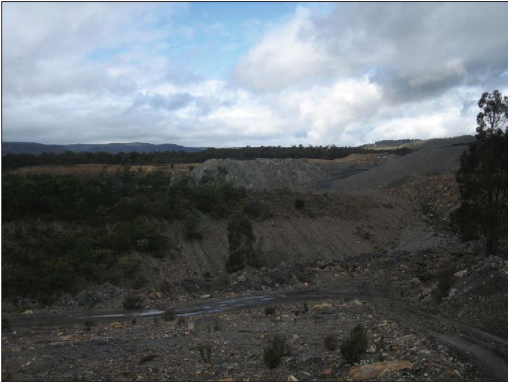
Plate 3-1: Lamberts North viewed from Mount Piper ash repository showing mining spoil and Huon Gully
