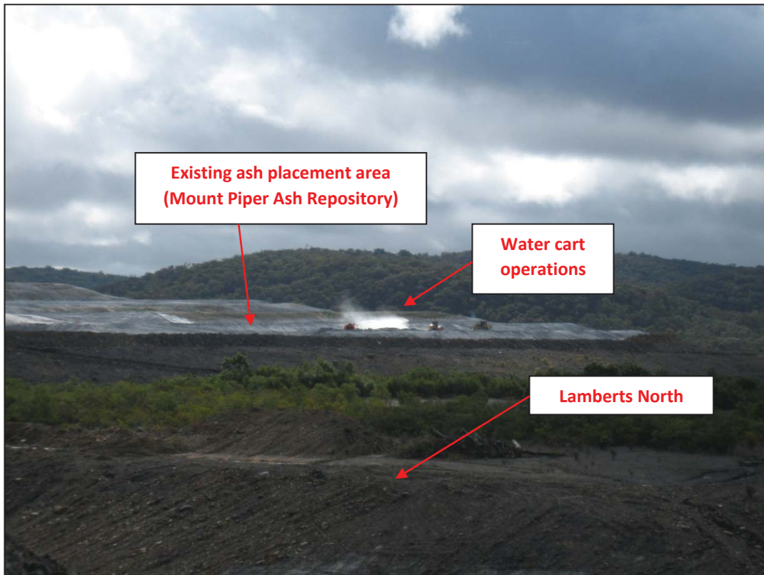
Plate 3-2: View from Lamberts North looking north-west across the revegetated mullock heap to the existing Mount Piper Ash Repository, showing water cart operations
