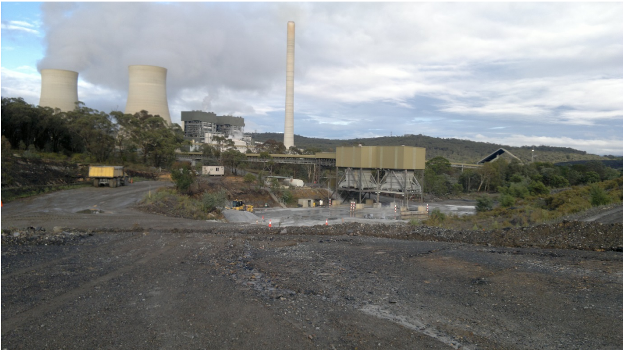
Figure 5 | Photograph of Lambert's North South eastern boundary near the bins
