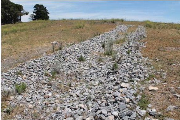
Water drop structure above SD5 in good condition and stable
