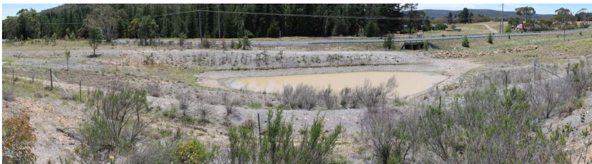
SD4 some rill erosion and bare ground during very dry conditions
