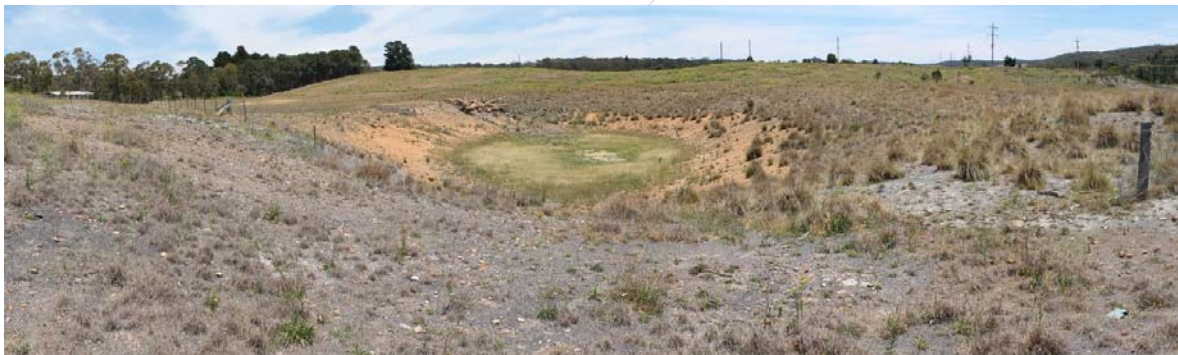
SD5 some rill erosion and bare ground evident during very dry conditions
