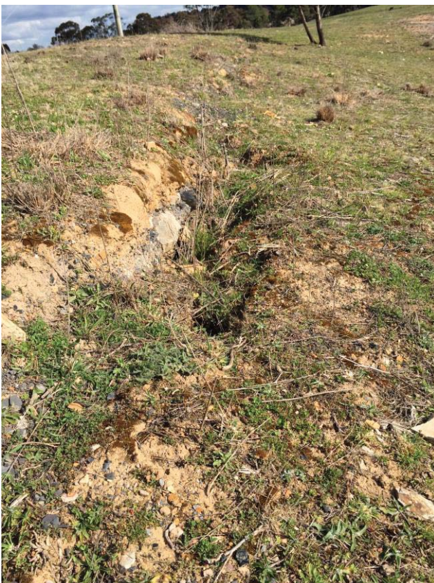
Figure 7 Example of soil cracking on slope crests
