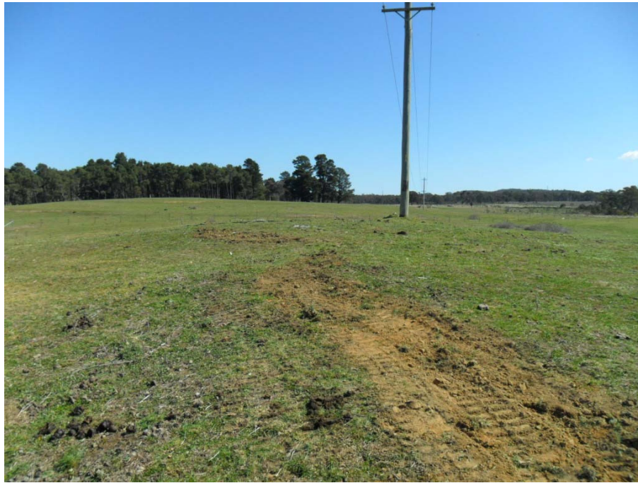
Plate 3 Cracking on crest of slope repaired
