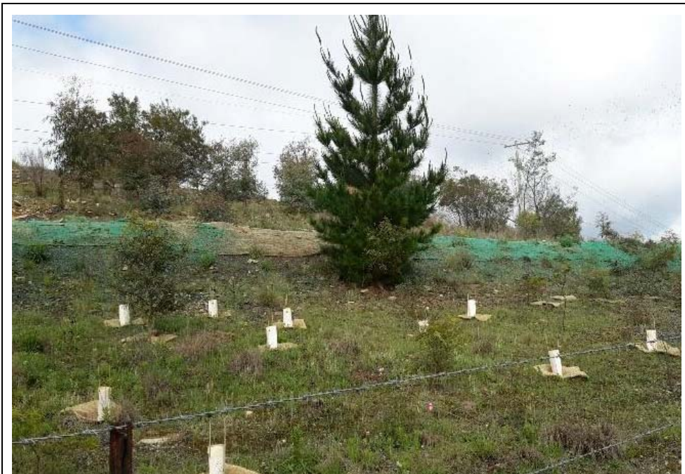
Plate 8 Tube stock planting, with jute mesh and hydromulch in background
