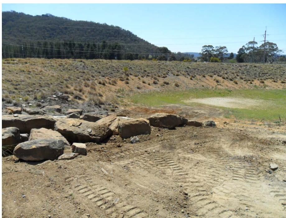
Plate 6 Sediment basin wall repair
