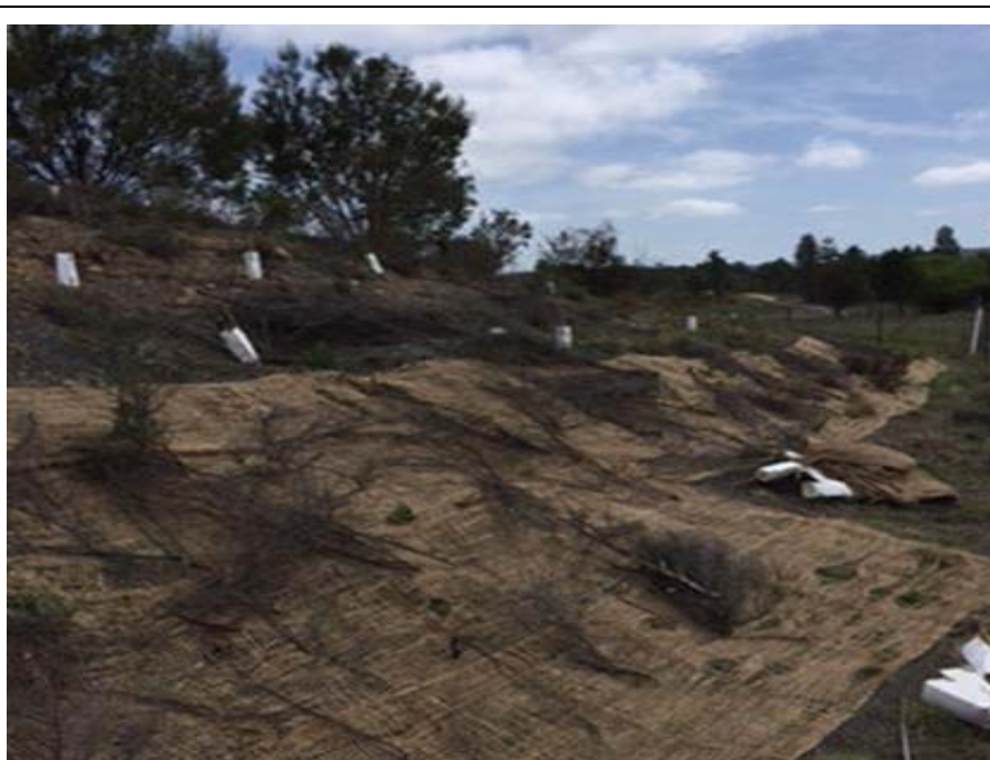
Plate 1 Jute mesh installation in treed rehabilitation area
