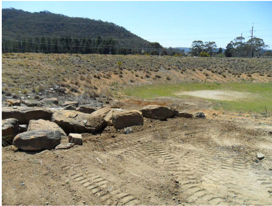
Plate 5 Sediment basin wall repaired
