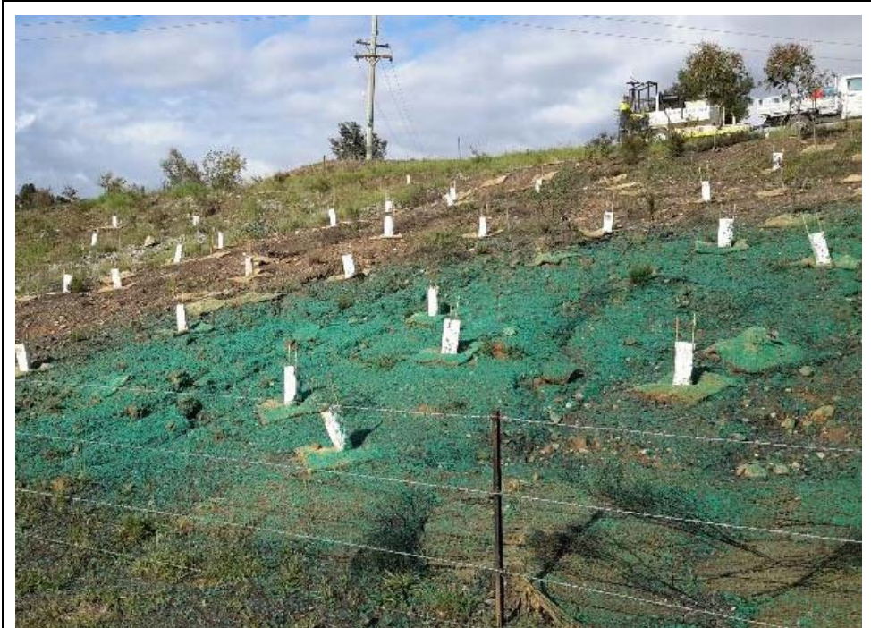
Plate 7 Hydromulch application in treed rehabilitation area
