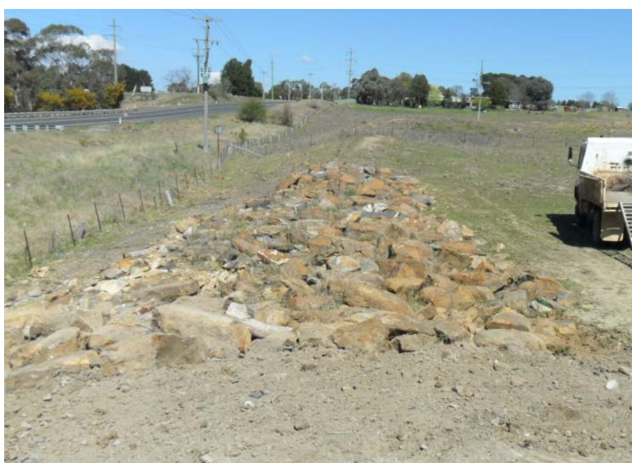
Plate 4 Repair to slope adjacent to Castlereagh Highway
