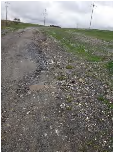
Figure 13 Rill erosion on main access trail
