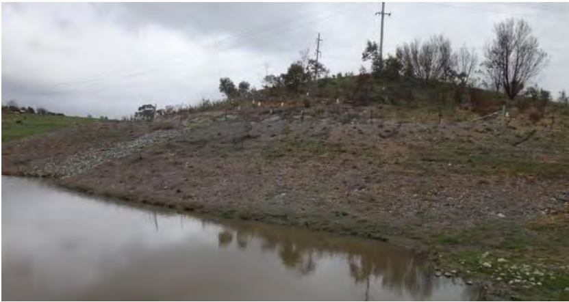
Figure 6 Sediment retention basin east of quadrat 2
