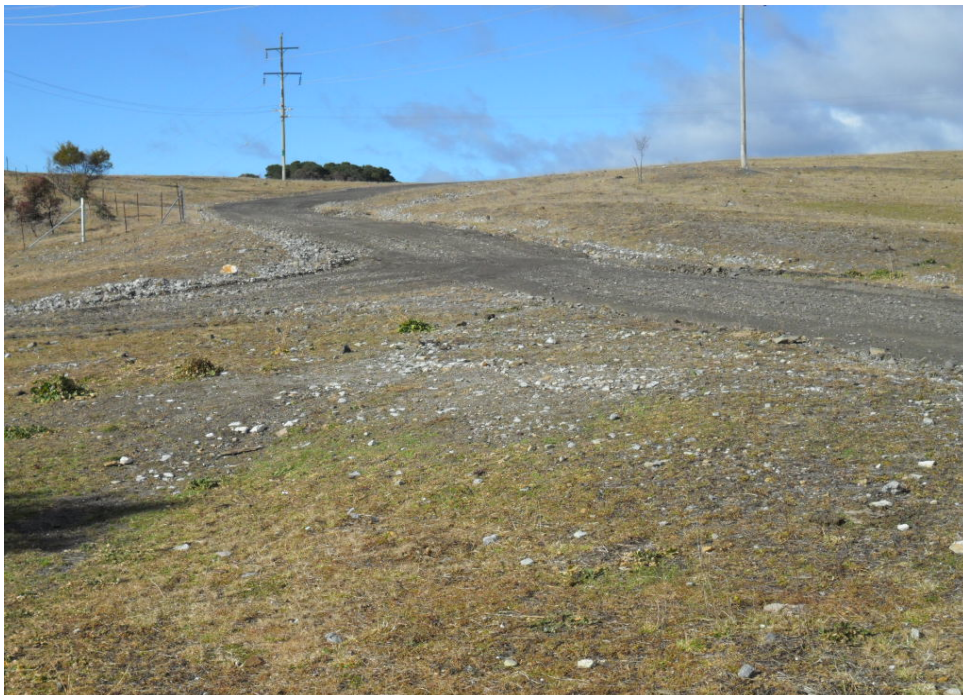
Plate 2 Access track grading – August 2017
