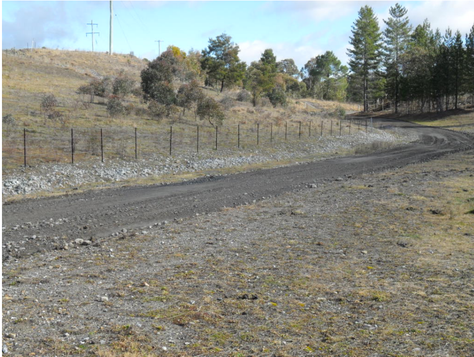
Plate 1 Access track grading – August 2017
