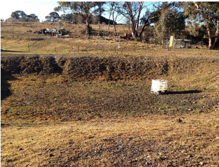
Figure 6 Sediment retention basin
