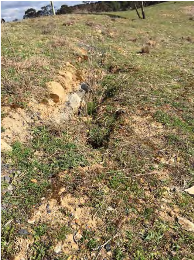
Figure 7 Example of soil cracking on slope crests
