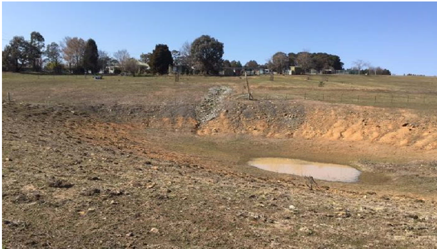
Figure 2 Indicative condition of sediment retention basins
