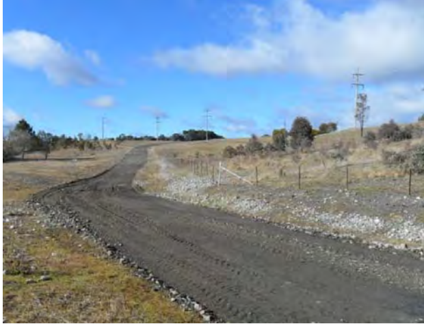
Figure 7 Recently graded trail
