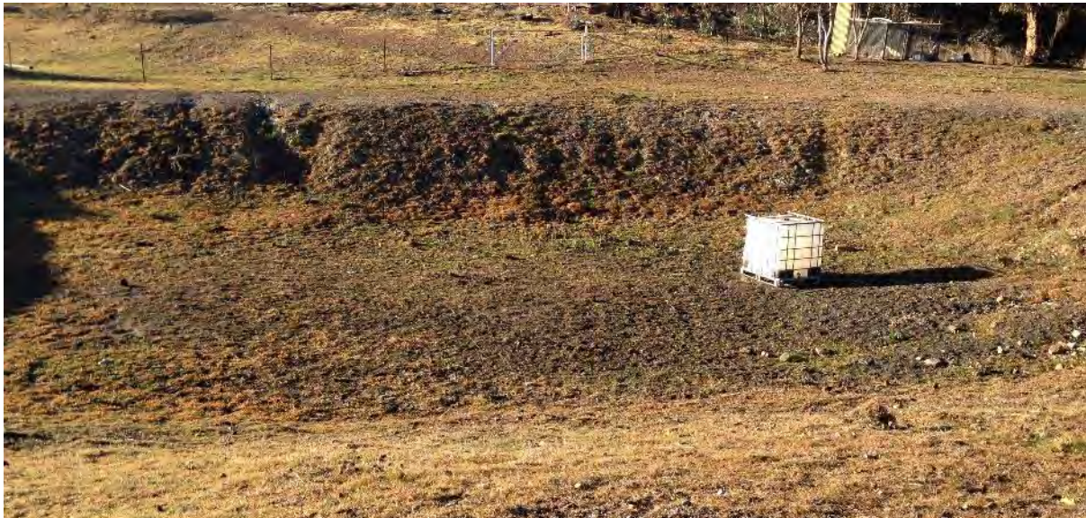
Figure 2 Indicative condition of sediment retention basins
