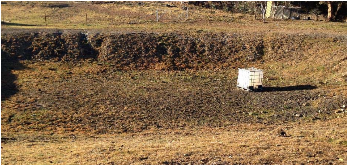
Figure 2 Indicative condition of sediment retention basins
