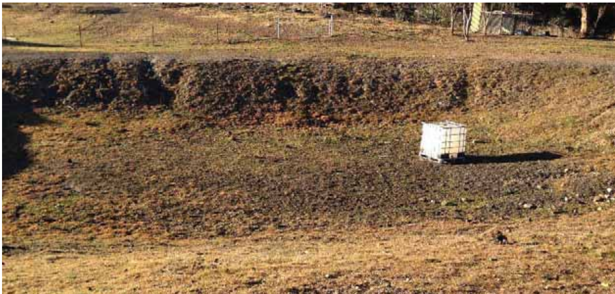
Figure 2 Indicative condition of sediment retention basins
