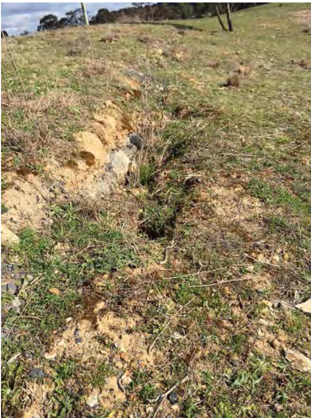
Figure 7 Example of soil cracking on slope crests
