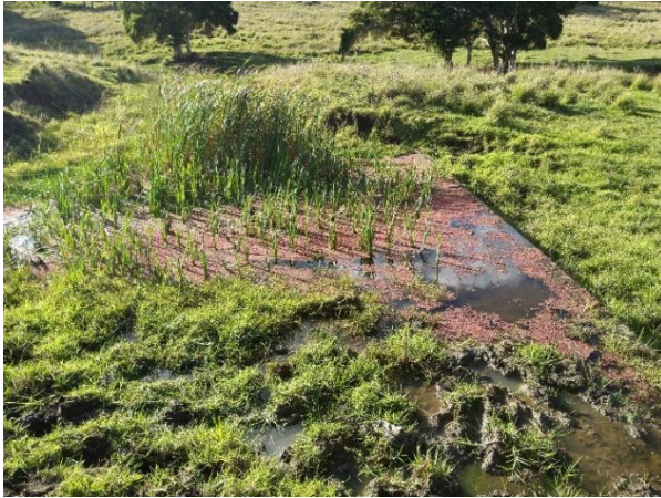
Figure 3-4 Bio-retention pond within drainage line
