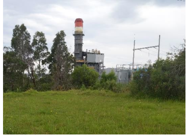
Figure 2-7 Acacia scrub within the switchyard car park area
