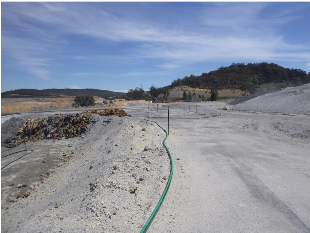
Photo 10 – Sprinklers and filter bags being disposed of at the ash repository
