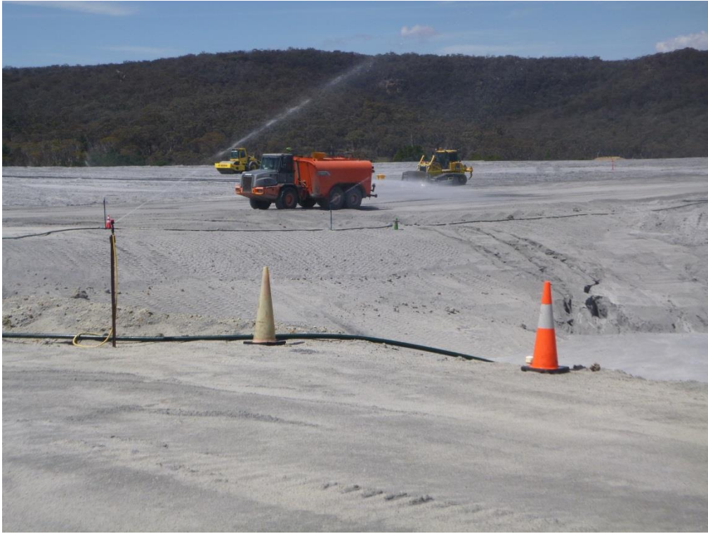
Photo 11 – Ash repository being compacted and sprayed by water truck
