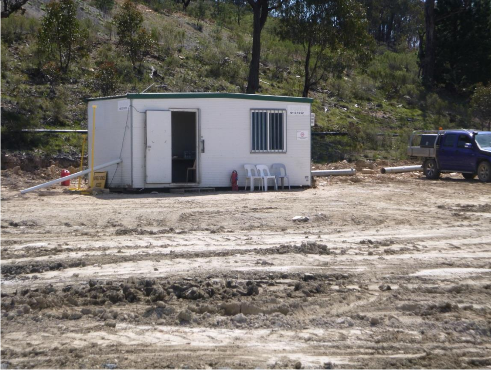
Photo 13 – Jerry can at the Lendlease laydown area. No visible waste or waste bins.
