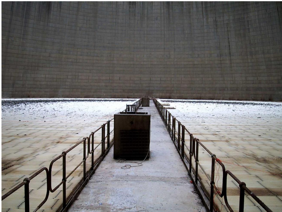
Inside one of Mount Pipers Cooling Towers
