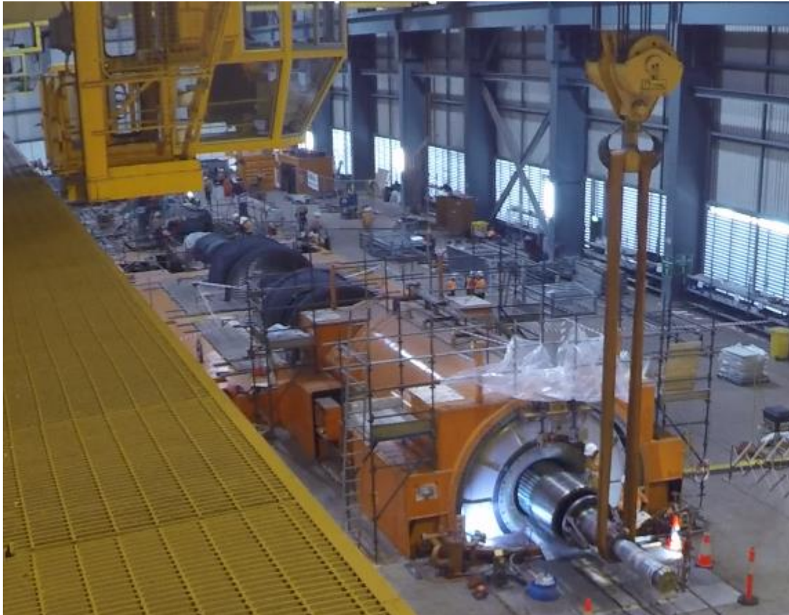
Mount Piper Unit 1 Turbine and Generator being Maintained
