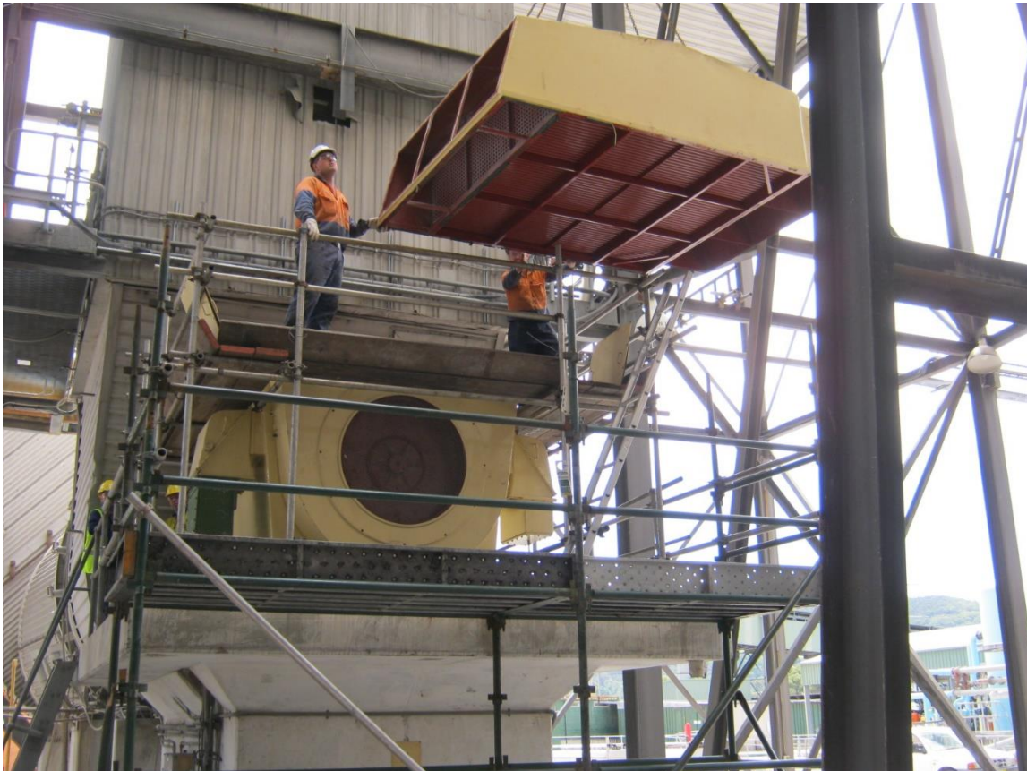
Disassembling and ID Fan Motor for removal
