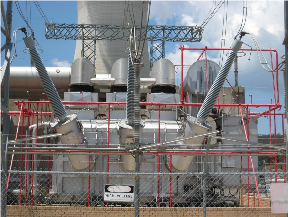
One of Mount Pipers Generator Transformers
