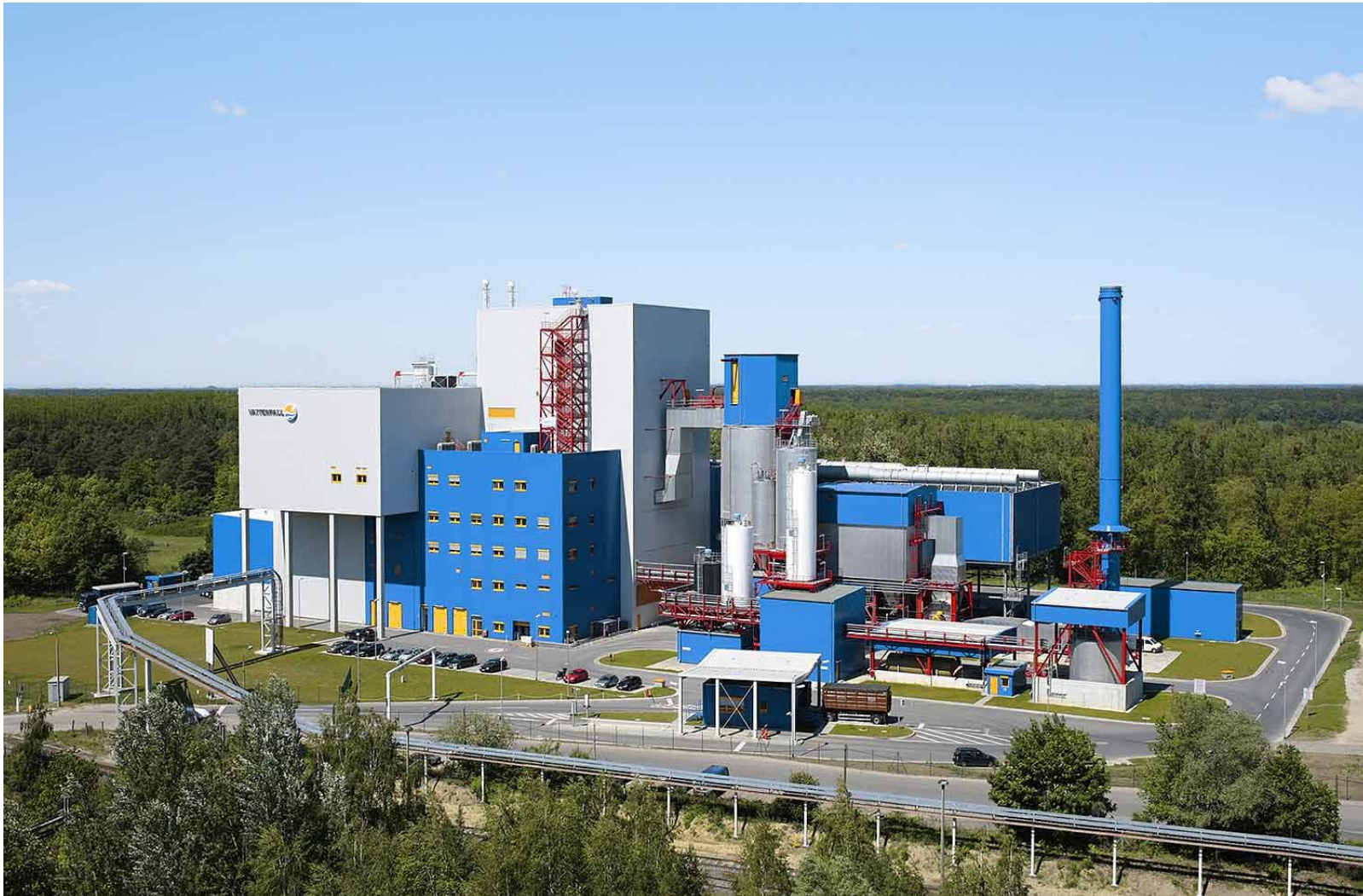
EfW in Rüdersdorf, Germany in operation since 2009
