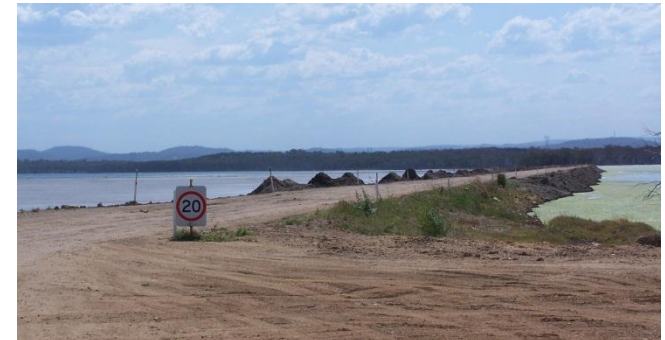
Ash Dam - raising pond 4 wall
