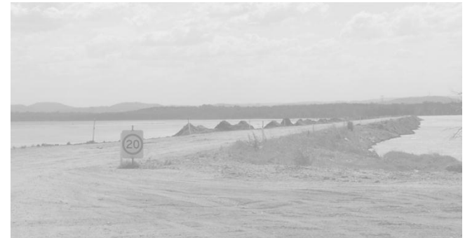
Ash Dam - raising pond 4 wall
