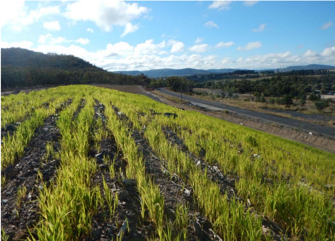
Photograph 7-1 Amenity Bund looking east following application of mulch and native mix 2015
