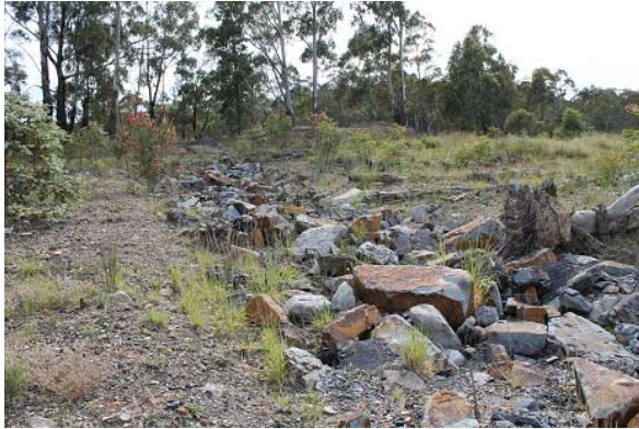
Area A: Stabilised water drop structure.
