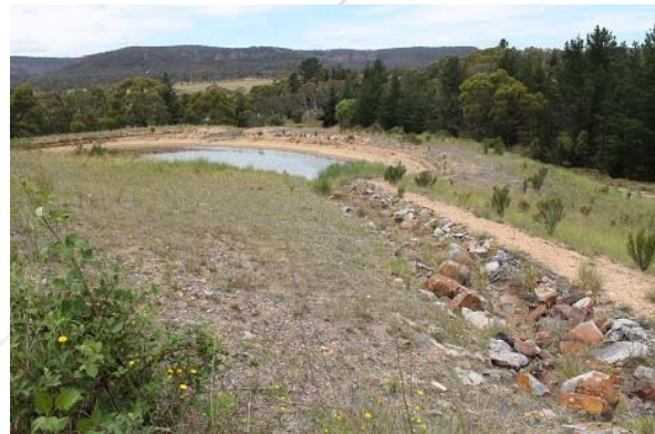
Area B: Stabilised water drop structure in good condition
