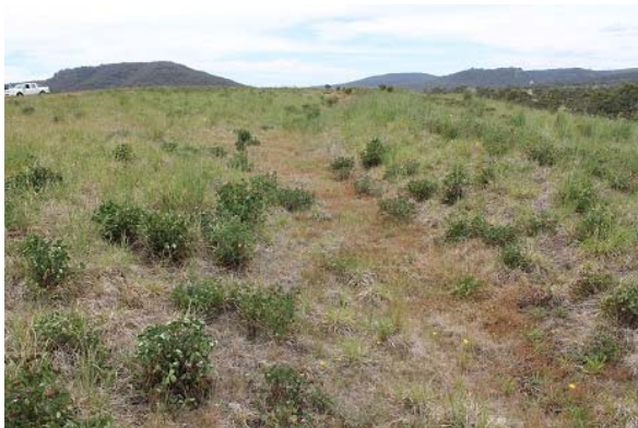
Area B: Stabilised contour drain with good vegetative cover.
