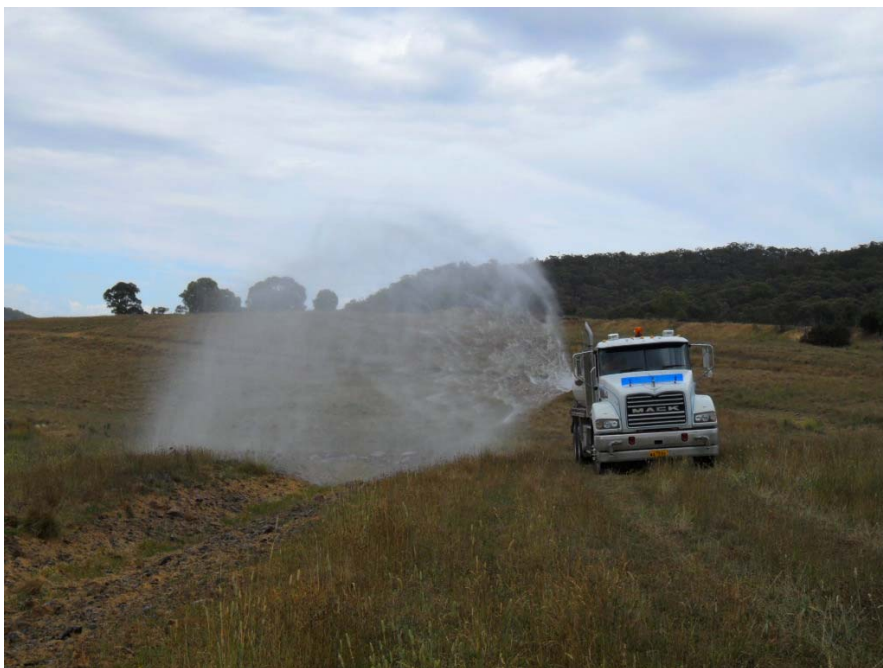
Plate 8 Area B & C – Watering of hydro-mulch drainage lines, December 2015
