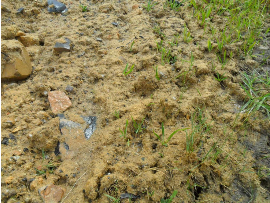
Plate 9 Area B & C – Germination of hydro-mulched drain, December 2015
