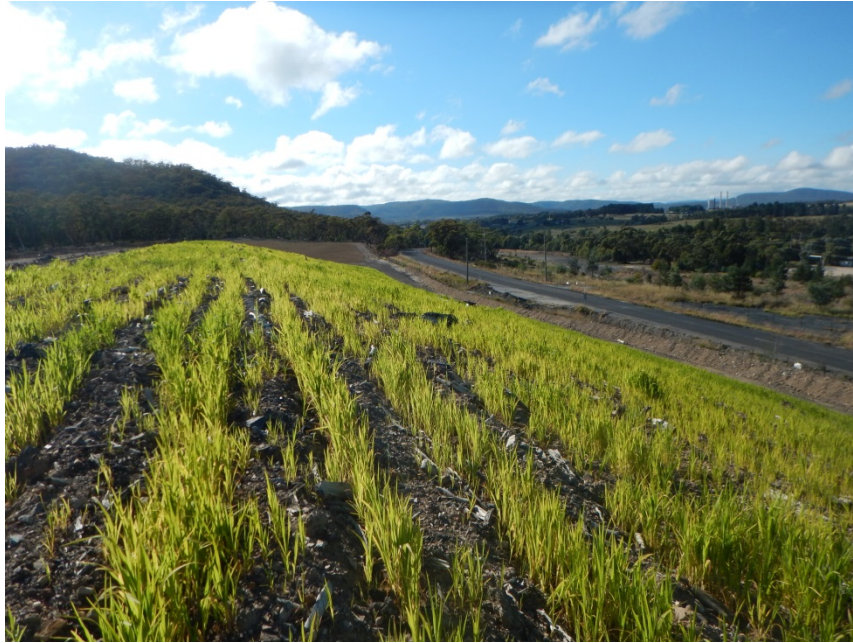
Plate 1 Amenity bund – application of mulch & native seed mix (2015)
