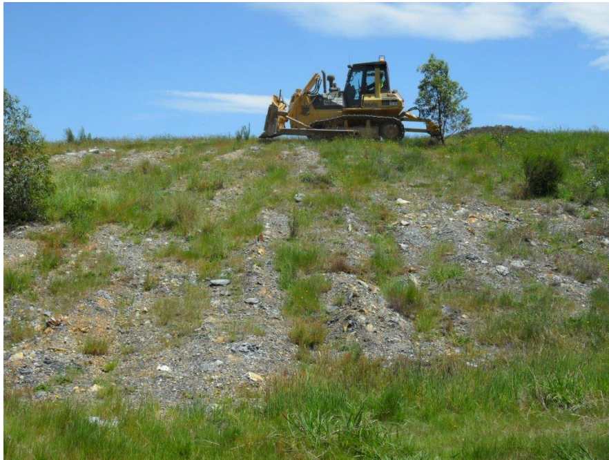
Plate 6 Area B & C – Mechanical ripping of poorly established pasture, November 2016
