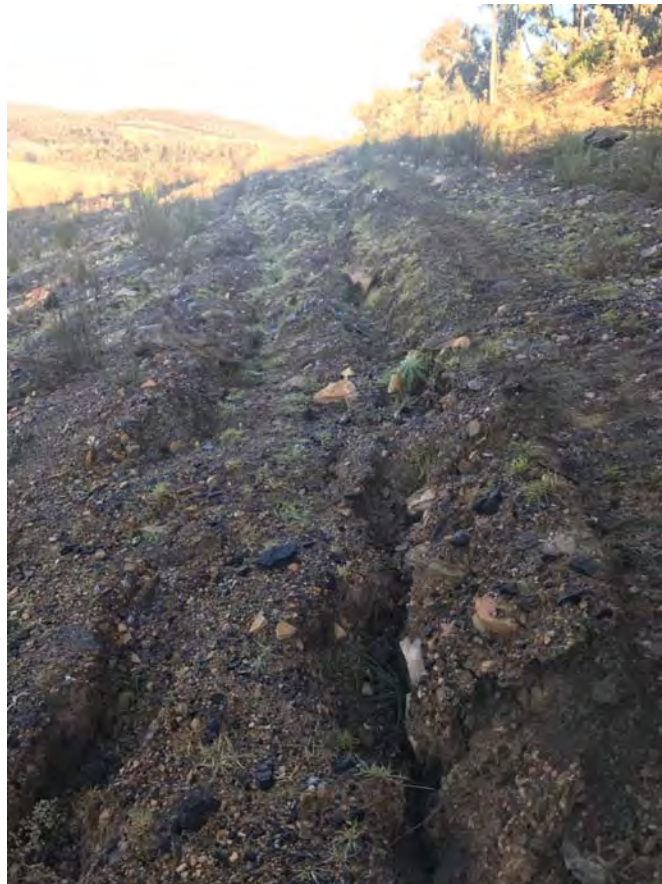
Plate 2 Surface cracking on slope in Yarraboldy Extension area, May 2017.
