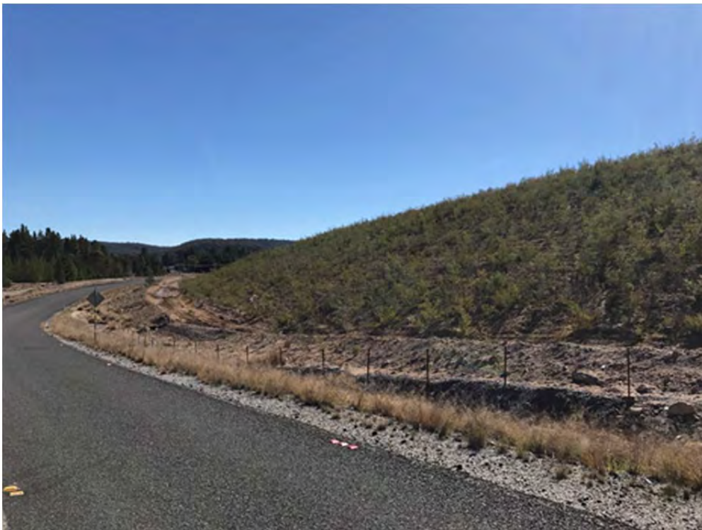
Plate 4 Repair of drainage line in Yarraboldy Extension area, June 2017.
