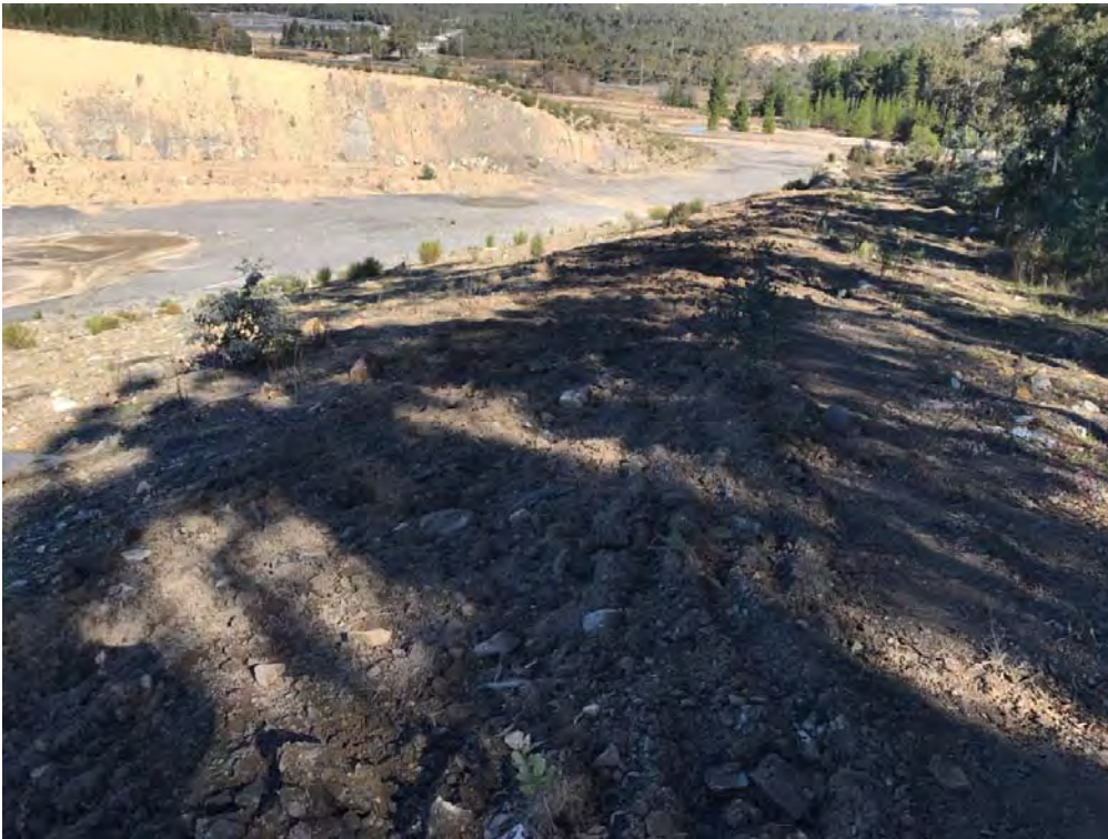
Plate 3 Repair of surface cracking in Yarraboldy Extension area, May 2017.
