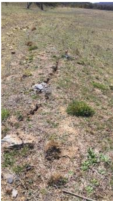
Figure 2 Extent of cracking along contour
