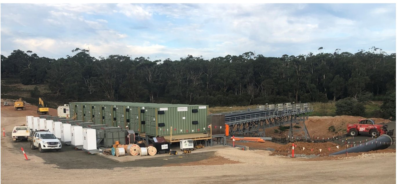
Cofferdam and Bypass Pump System construction continues
