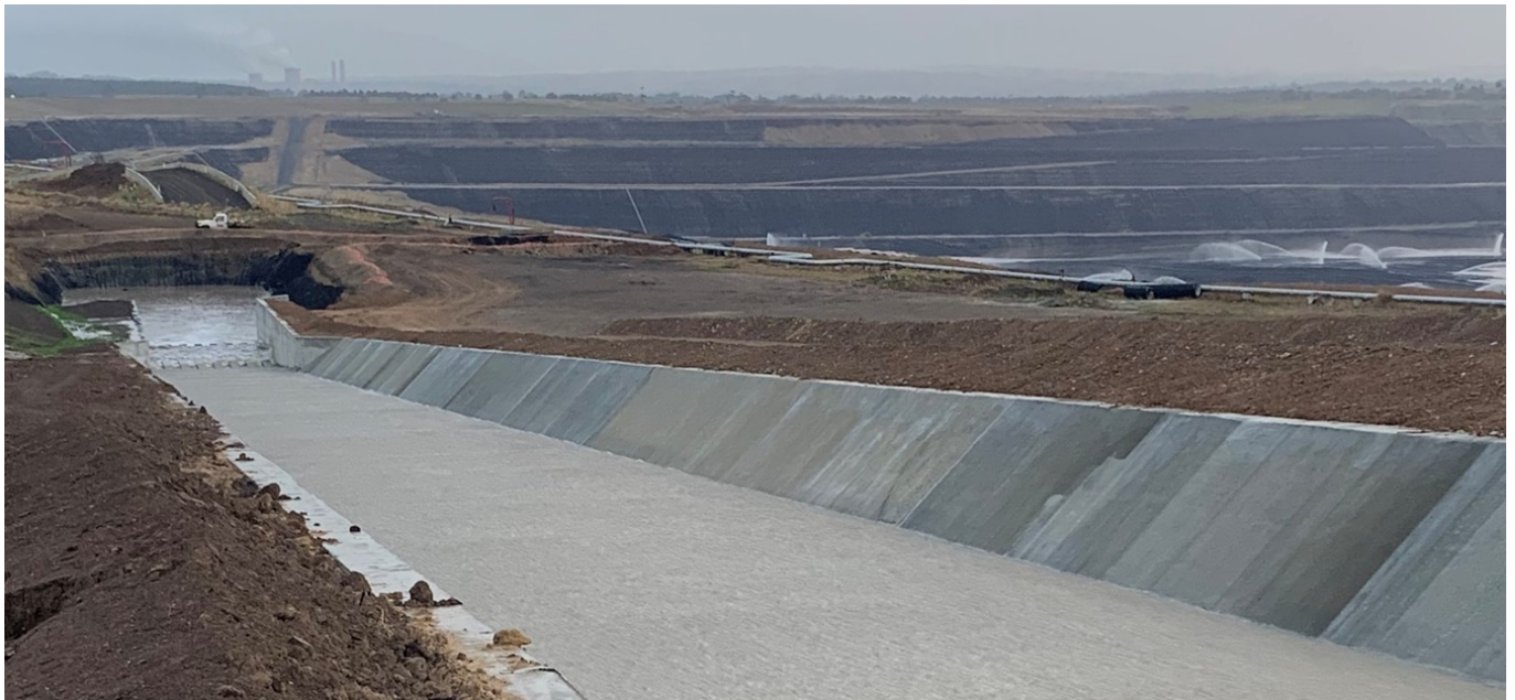
Engie diversion completed and activated 4 March 2022
