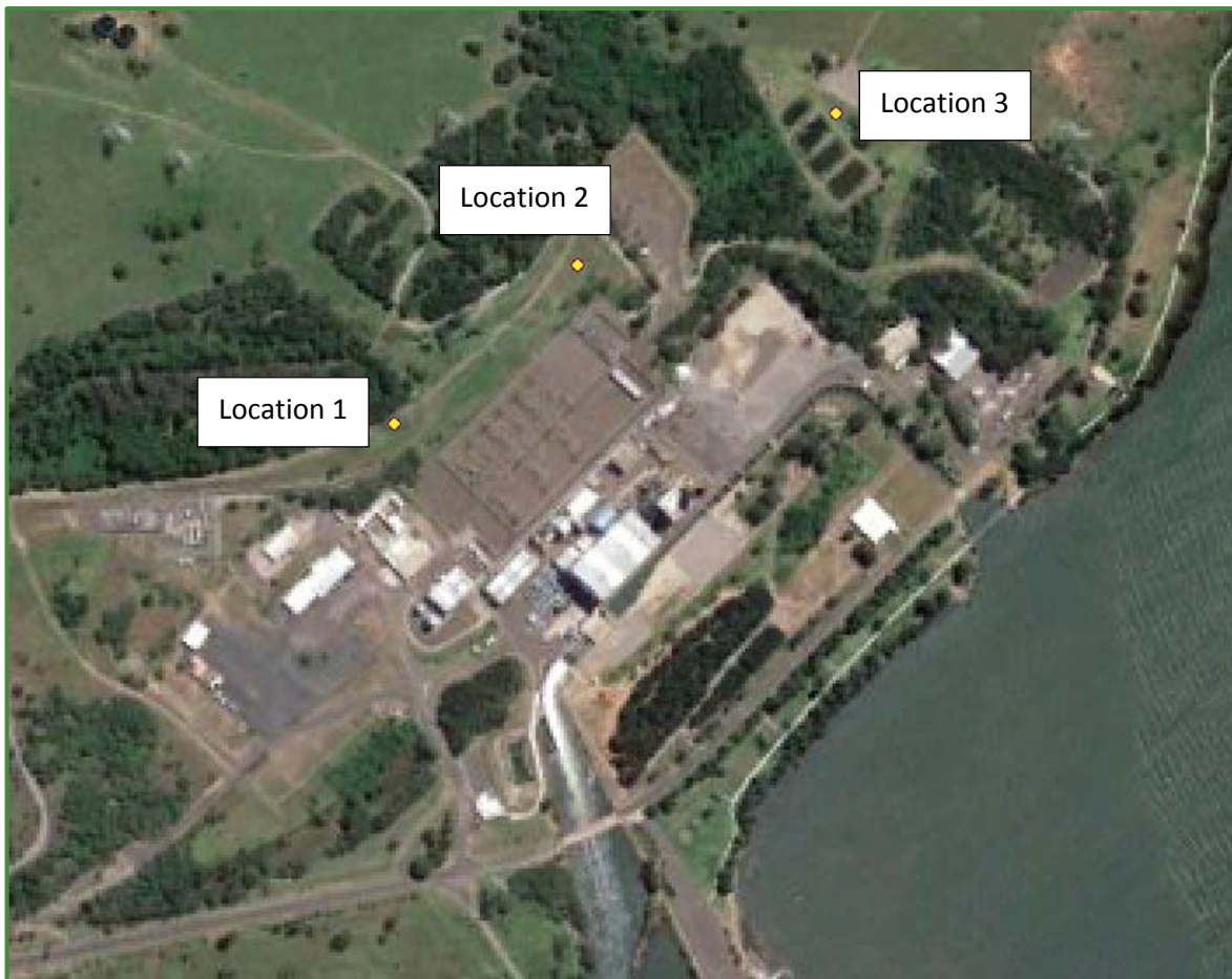
Figure 3-2: Existing Plant Noise Measurement Locations
