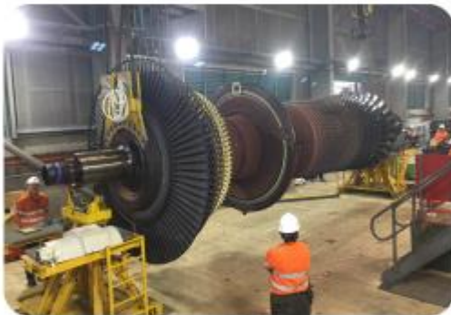
The main turbine at Tallawarra A during maintenance
