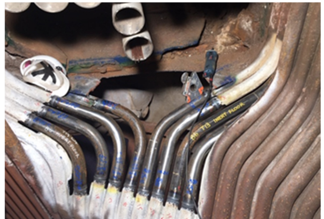
Replacing corroded sections of the boiler burner tubes
