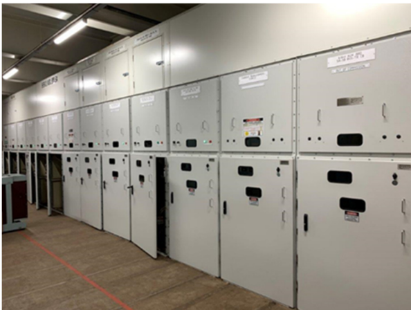
Works completed as part of the Arc Flash upgrade
