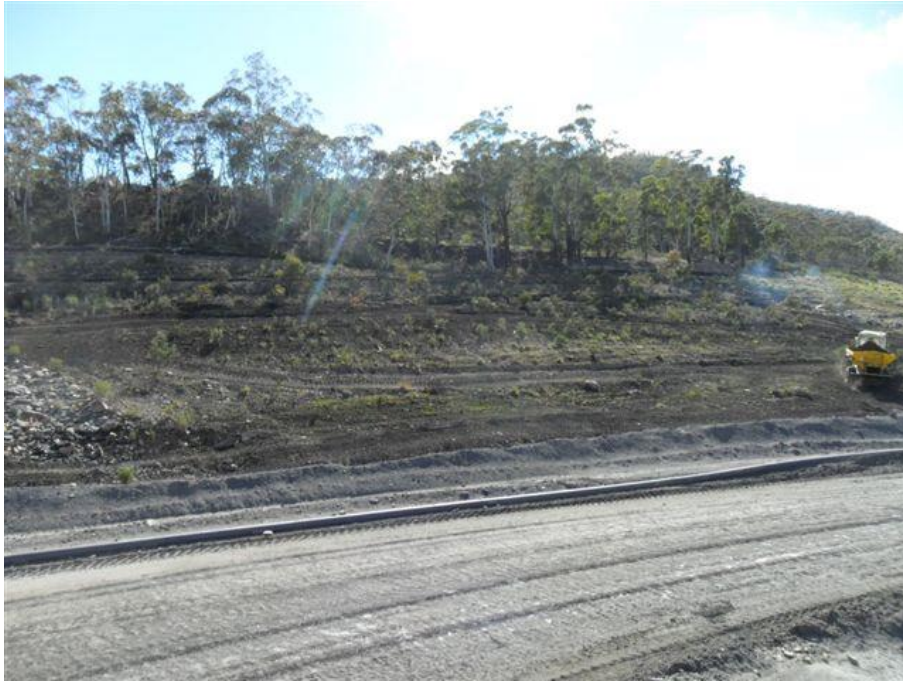
Plate 2 Area A Rehabilitation Looking North East during mulching process
