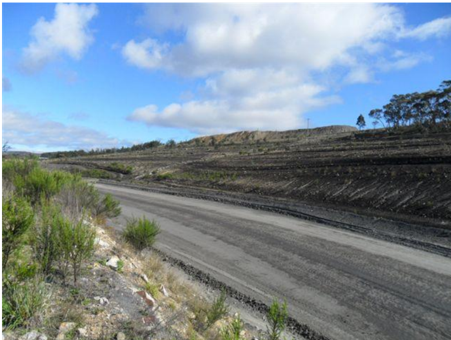
Plate 3 Area A Rehabilitation Looking North
