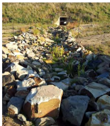
Plate 2 Rock lined drainage line in rehabilitated area C
