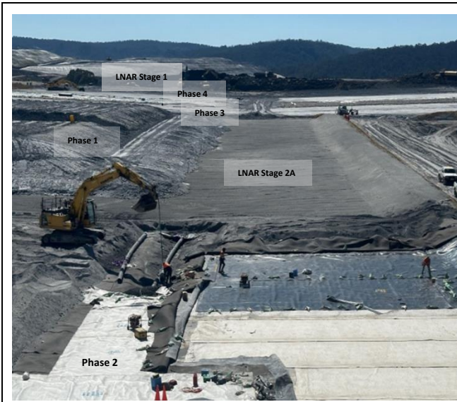
Plate 3 Linear Pipework Installation at LNAR Stage 2
