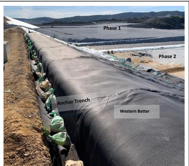
Plate 4 Installation of Linear
