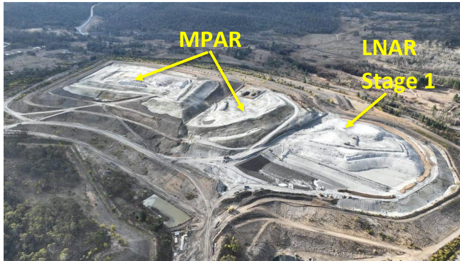
Plate 2 Aerial view of Mount Piper Ash Repository (MPAR) and LNAR Stage 1 (A and B) areas (Photo taken 16 August 2023)
