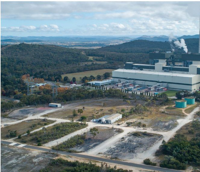
Location of the Mt Piper BESS.
